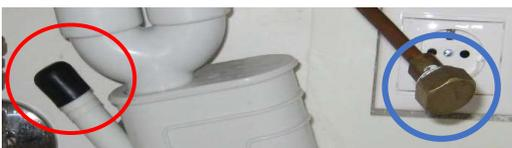
Picture 1. The dishwasher drain hose plug (plastic) and water intake line plug (brass)
