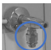
Picture 2. The washing machine water supply hose plug
